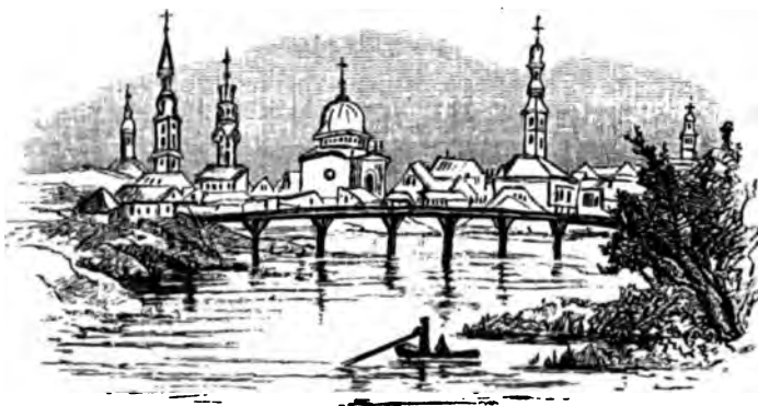
From the bridge which crosses the Kőrös, a good view is obtained of the town with its glittering steeples of black
